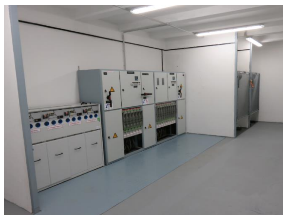
Figure 57: TS Moša Pijade, Maribor after reconstruction
