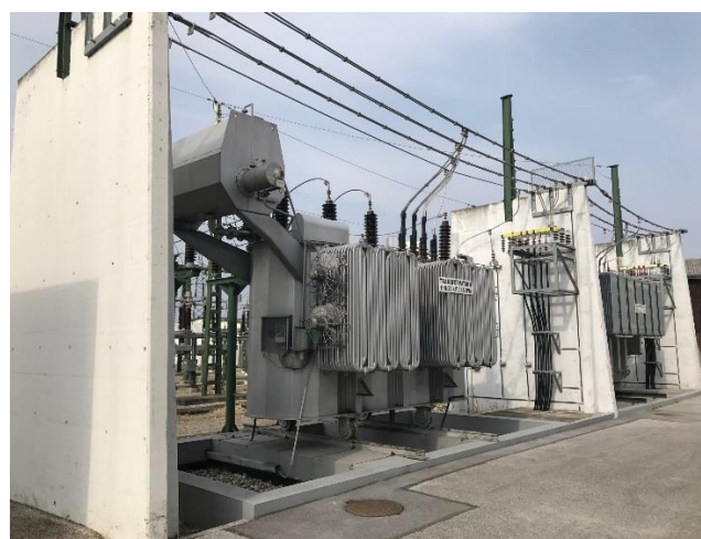
Figure 52: 110/20 kV Ljutomer STS
