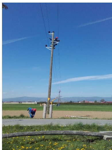
Figure 54: Reconstruction of the Cirkovce–Pongrce–Gaj power line
