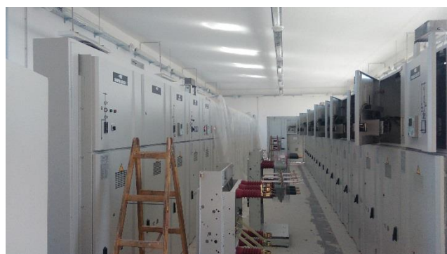
Figure 50: 110/20 kV Slovenska Bistrica STS - 20-kilovolt switchyard
