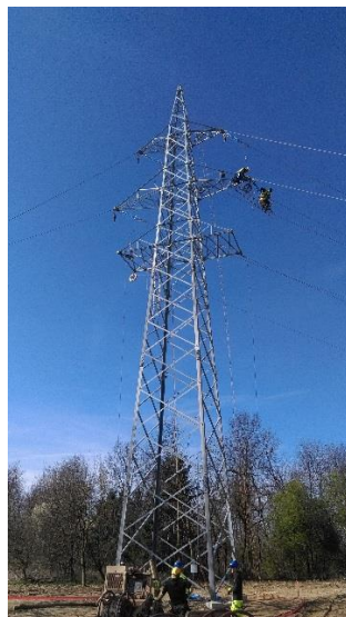
Figure 49: 2 x 110-kV Murska Sobota–Mačkovci power line
