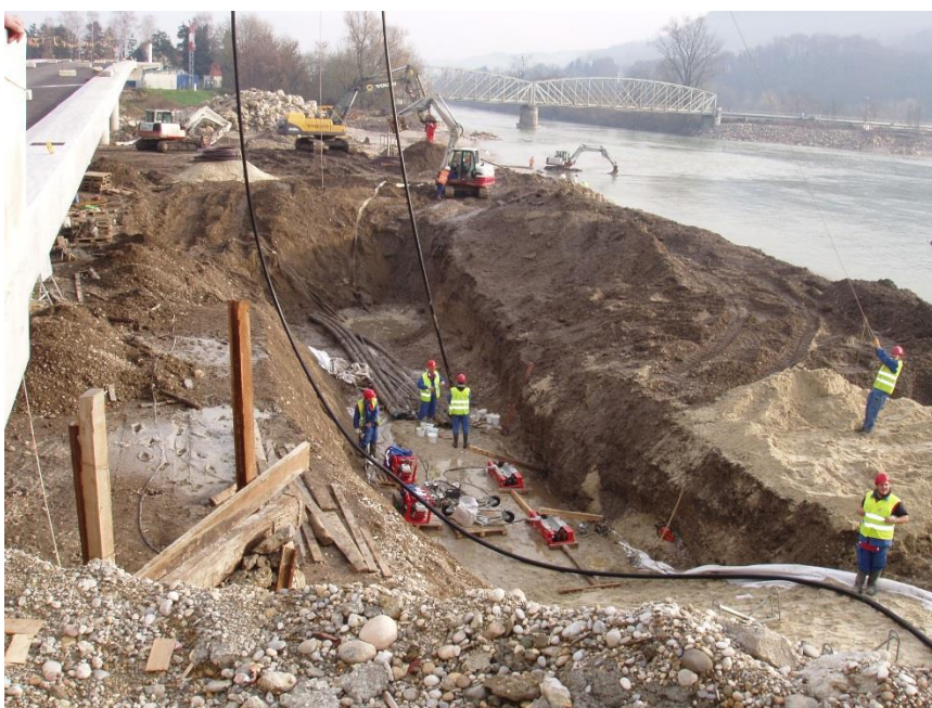
Figure 62: Execution of works on the 110 kV cable lines for the needs of the hydroelectric power plant on the lower Sava
